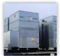
Packaged forced draft counterflow cooling tower
