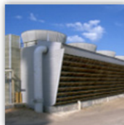
Field erected induced draft crossflow cooling tower
