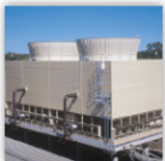
Field erected induced draft counterflow cooling tower
