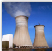
Field erected natural draft counterflow cooling tower
