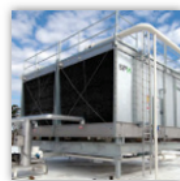
Packaged induced draft crossflow cooling tower
